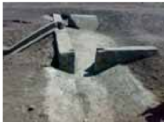
Figure 4.7: Drop structure with 2 off-takes, but without gates installed yet
