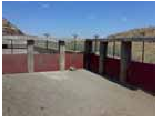
Figure 4.4: The sluices and rejection spillway
